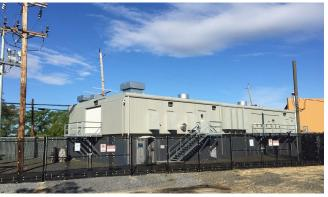
Post-Sandy, the MTA reconstructed and raised substations along the Long Beach Branch.
