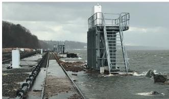
Elevated equipment platforms protect critical equipment during flooding from a combination of high tide and storm surge on January 13, 2024.
