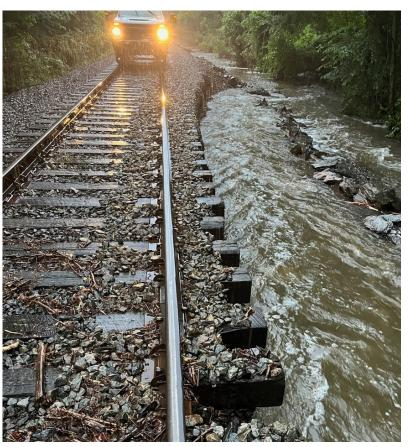
Track washout south of the Dover Plains Station after heavy rain and flash flooding on July 10, 2023.
