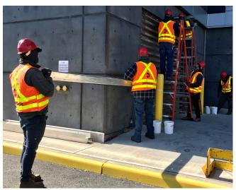
Deployment testing of flood logs at Clifton Shop, March 2023.
