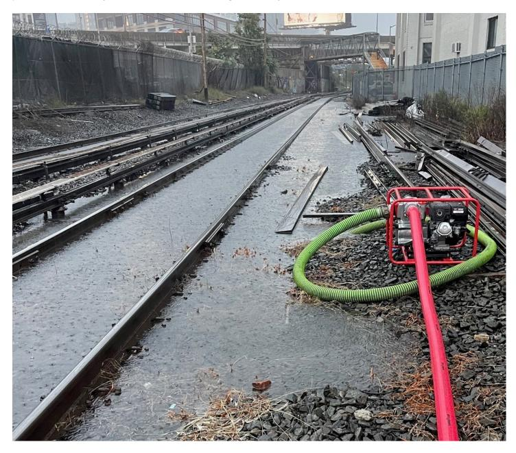
Portable pumps deployed to mitigate torrential rainfall flooding near Hunterspoint Ave right-of-way during Tropical Storm Ophelia, September 29, 2023.
