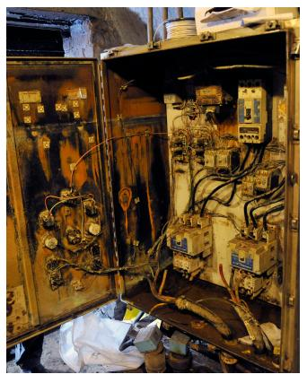
Corroded and damaged electrical circuits following Superstorm Sandy, 2012.
