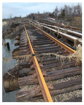
Washout, corrosion, and damage on the Rockaway Line A S, following Superstorm Sandy, 2012.
