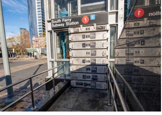
Testing of coastal surge flood logs installed post-Sandy at the South Ferry Station 1 elevator.
