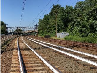
Application of heat reflective white paint along a curved section of rail near Rye on the New Haven Line.
