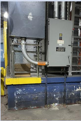
Elevated electrical equipment inside Castleton Depot. Electrical equipment in Castleton Depot is elevated above flood depth to reduce the likelihood of major damage in the event of future floods.
