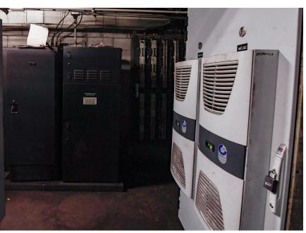
Self-cooling data cabinet in the communications room at the Wall St Station on the Lexington Avenue 4 5 Line.
