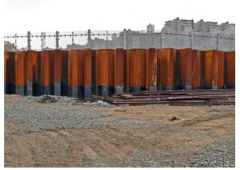
The Coney Island Yard perimeter flood wall under construction, October 2019. The perimeter flood wall, now complete, spans 12,000 linear feet and is driven approximately 30 feet below ground.
