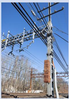
Catenary system counterweights help the system adust to temperature fluctuations.
