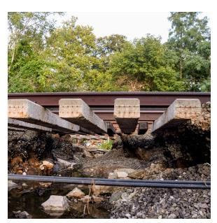
Flooding from Tropical Storm Ida washed out a culvert and the ballast supporting tracks at Dobbs Ferry, September 2021.
