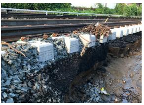
Washout from torrential rainfall flooding near Bayside on the Port Washington Branch from Tropical Storm Ida, September 2023.
