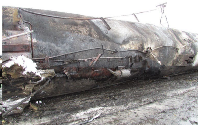
2(d) Bottom, showing fire damage and bottom outlet.
