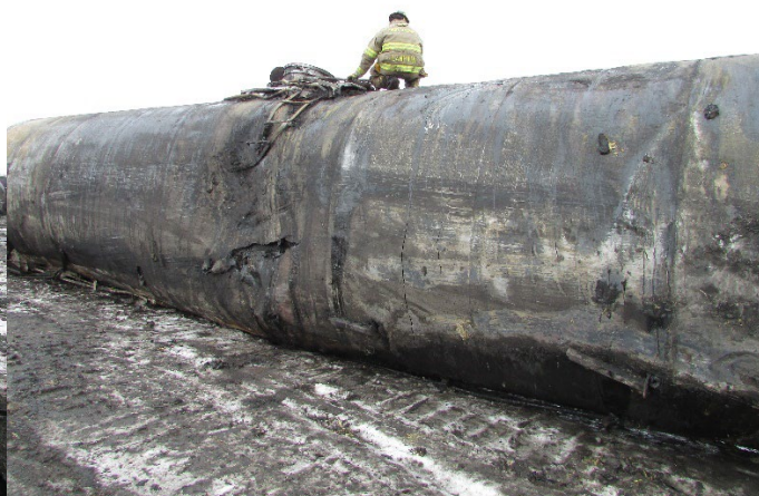
3(d) Left side of car from A-end showing damage to heat shield.
