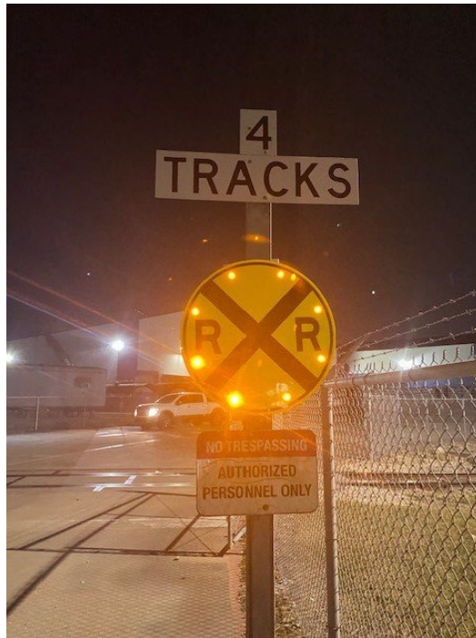
Figure 5. Highway-railroad grade crossing signage with LED lights.
