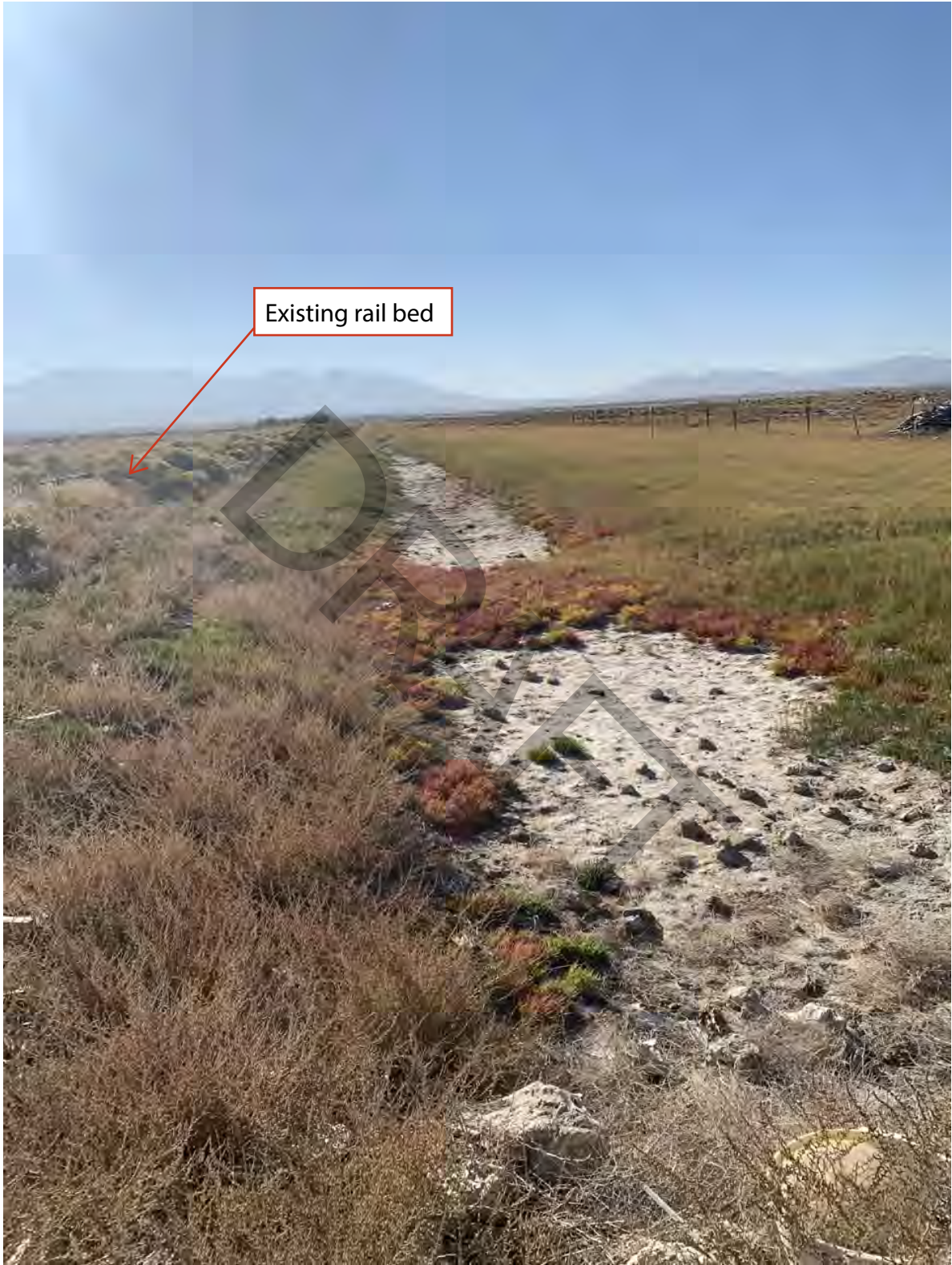
Typical wetland ditch along west side of rail line
