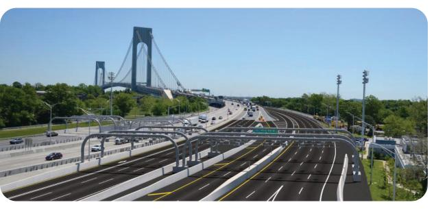
Figure 25 Toll gantries (the arched metal structures over the roadways) at the Verrazzano-Narrows Bridge
