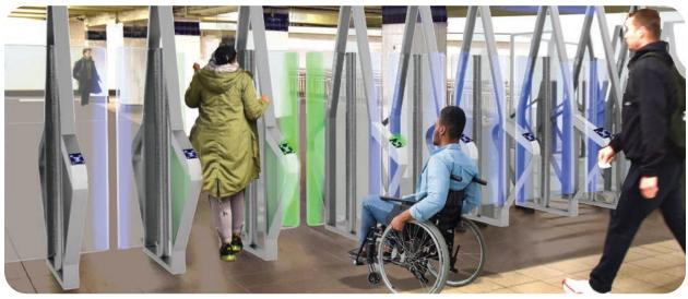
Figure 17 Rendering of double-door faregates at Jay Street station showing ADA functionality.
