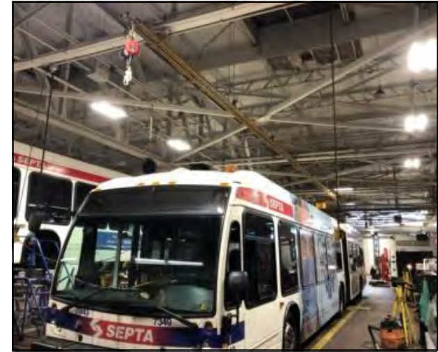
Maintenance Shop Equipment—Fall Arrest System
